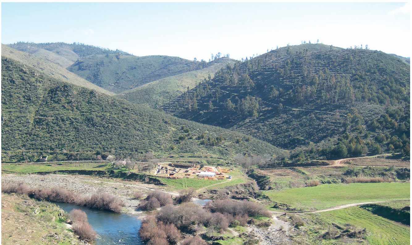
FIG. 2. — Right bank excavation overview.
